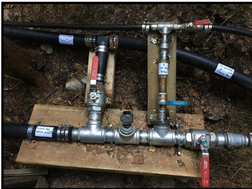
Figure 4. Water system. Excellent example of a water system designed to get water to sprinklers. All of these features are available locally.
